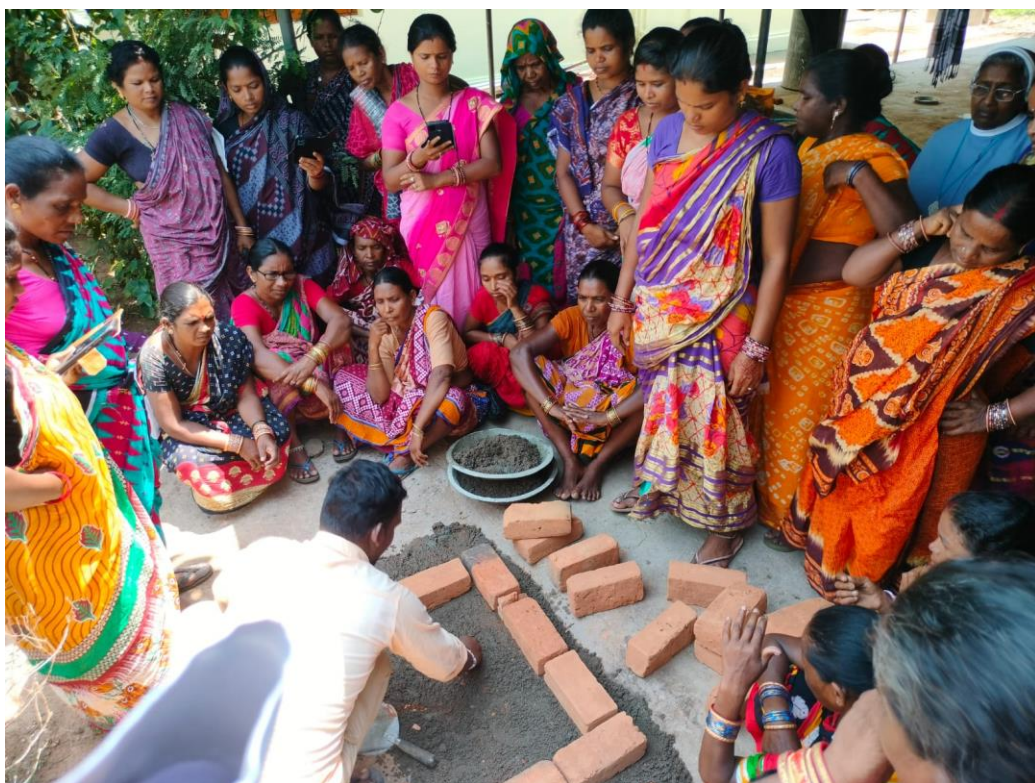
Training of 3 batches of women for five days on how to construct a smokeless chulha
