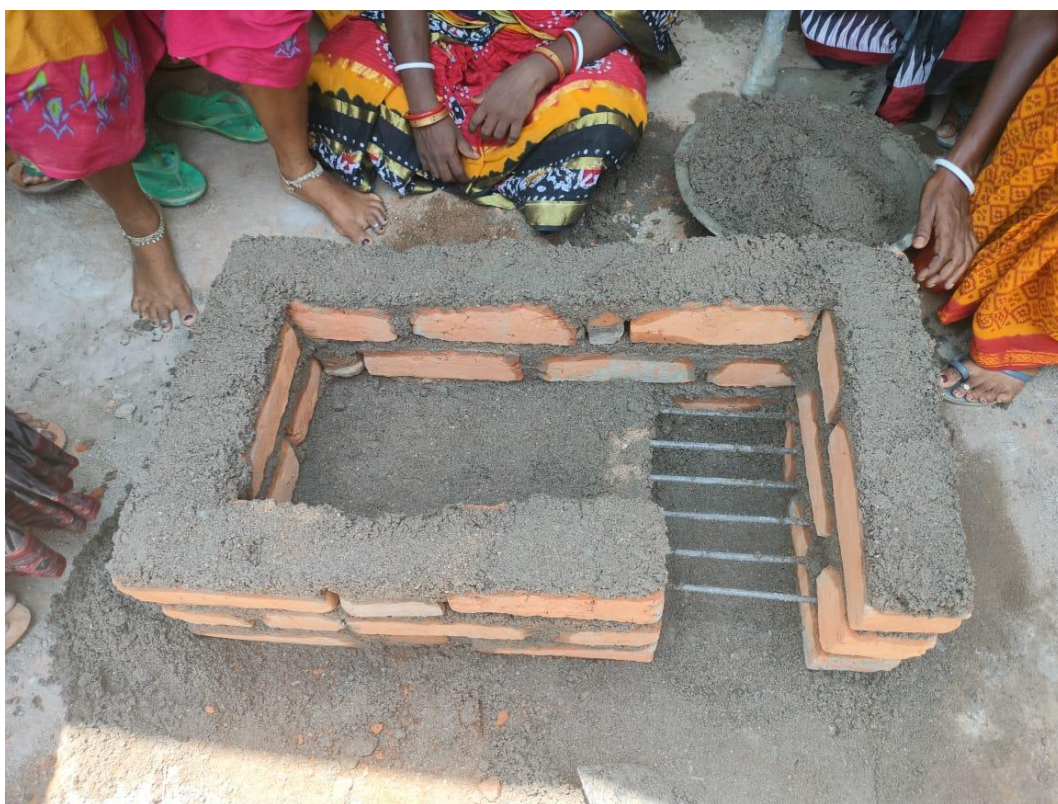
Training of 3 batches of women for five days on how to construct a smokeless chulha
