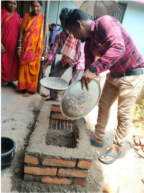
Training of 3 batches of women for five days on how to construct a smokeless chulha
